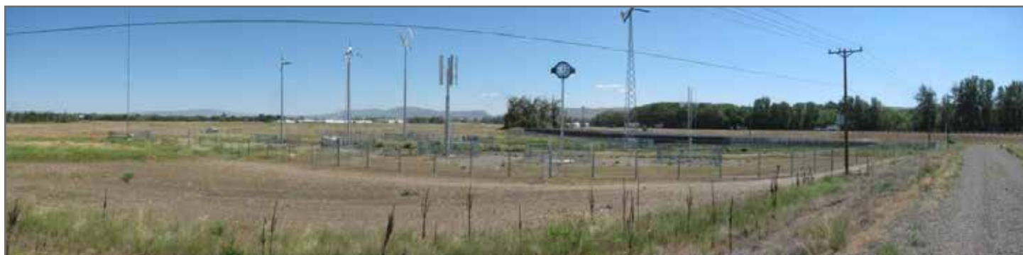
The City of Ellensburg tested solar panels and wind turbines.
